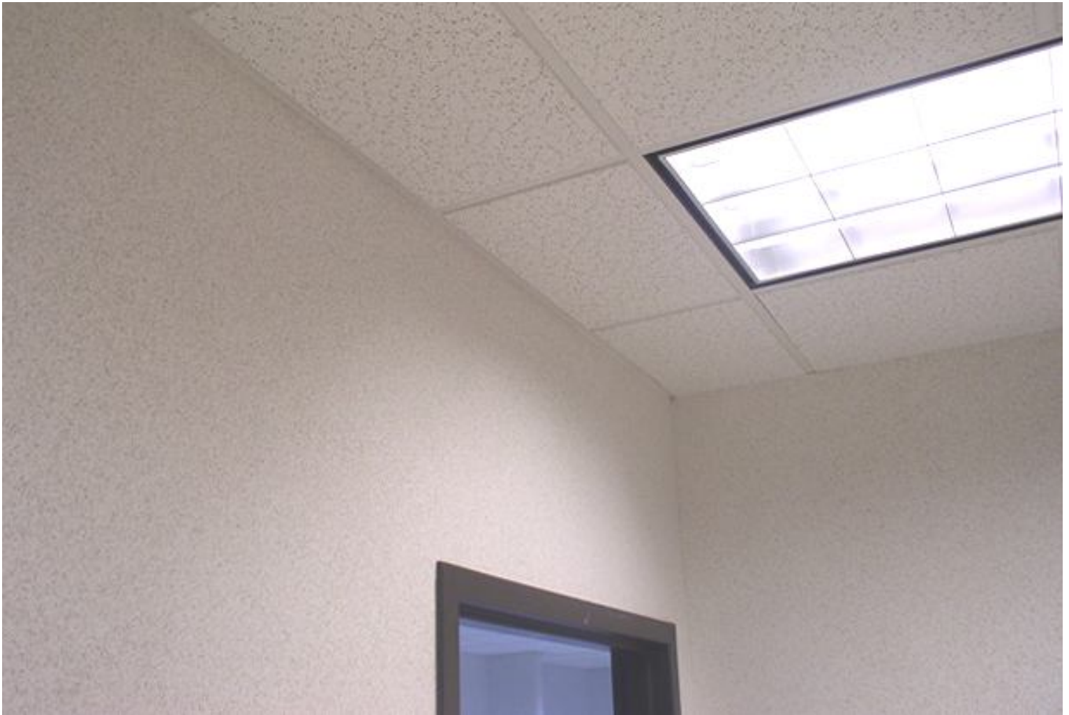
Eliminator Track at finished wall and acoustical ceiling.
